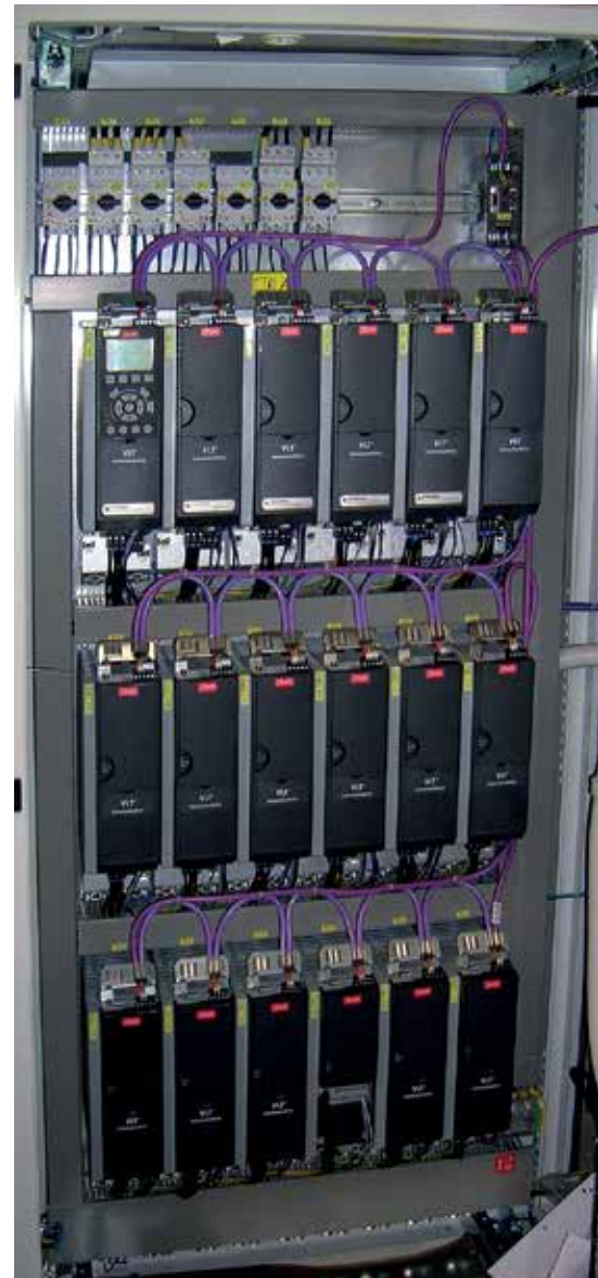
Variable Frequency Drives can be installed centrally (in a cabinet) or locally (close to the motor). Both options have advantages and drawbacks.
